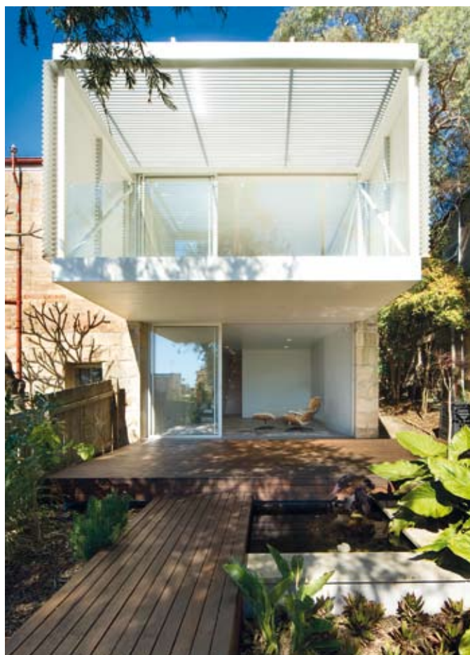
The rear deck cantilevers over 3m into the garden. PHOTOGRAPHY JOHN GOLLINGS
